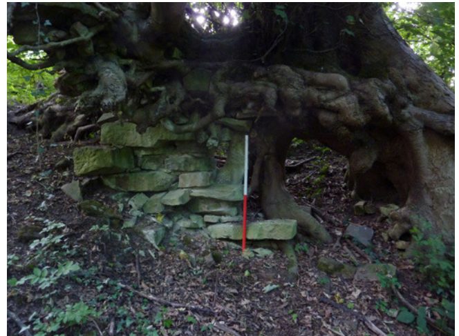
Wall remains at rear of engine house
