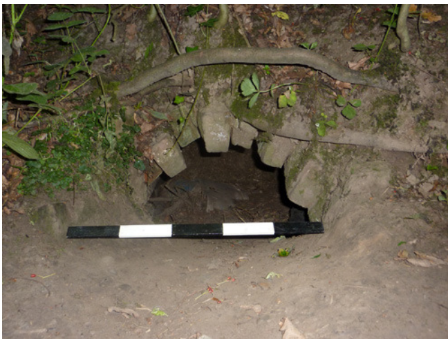
Flue to chimney
